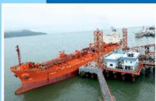
New Third Chemical Berth
