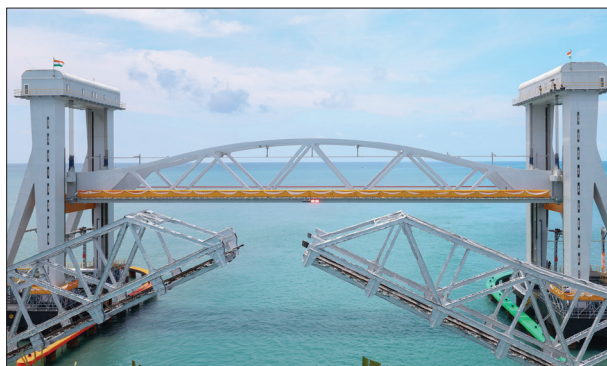
Pamban Bridge's 72.5-metre-long, vertical-lift span, a first for Indian Railways, makes it special.
